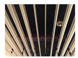
Above: Strand SS Ebony as primary ceiling (sound absorbing) above the metal baffles (visual lines for aesthetics)
